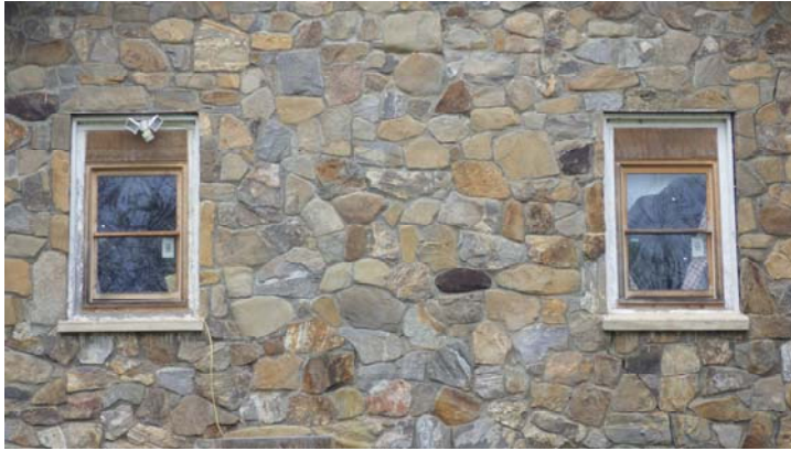
Replacement Windows on the Rear
