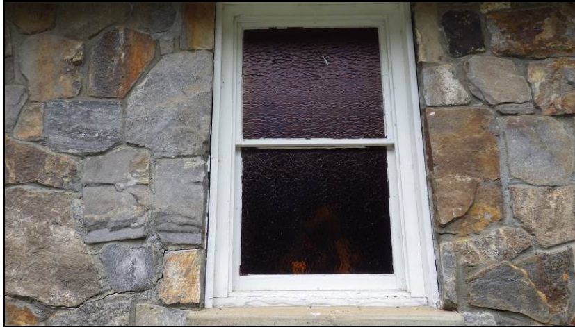
Original, one-over-one, double-hung wood sash window with textured pane
