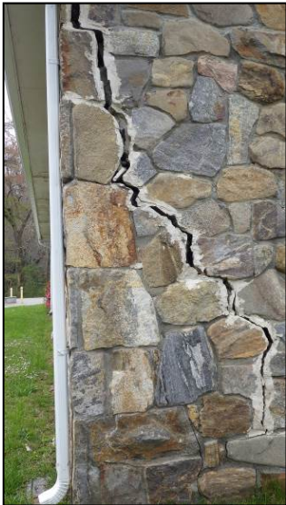
Structural Cracking
