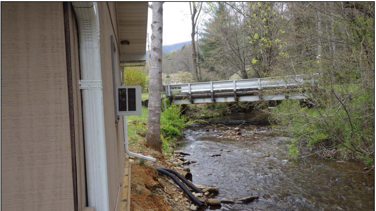
Westerly View toward Bridge No.127, from the North Elevation of Mount Sinai Church (MA0334)
