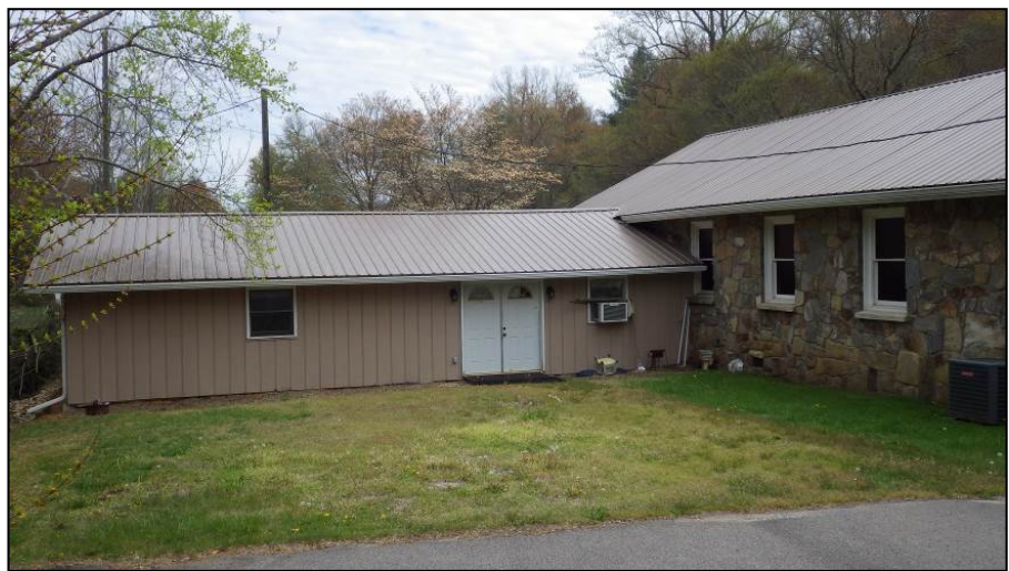
Northeast Addition (c.1970)
